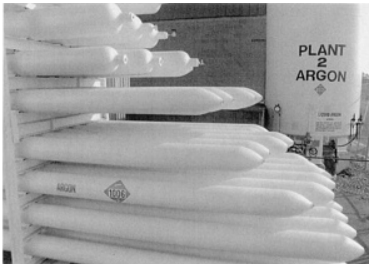
Fig. 5 Liquid argon storage and tube bank storage for argon gas. Courtesy of Bodycote IMT, Inc.
